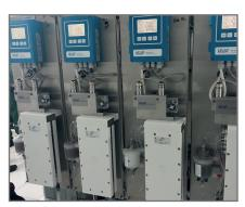
Feedwater monitoring is of highest importance in water steam cycles, where availability and reliability of continuous online measurements is critical.
